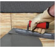
Ash Grove Pro® Skim Patch is a trowelable Portland cement based patching compound for use as a quick-setting floor underlayment.
